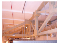
Customized Indoor Fire Structure Protection
