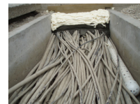
Cable Trough Sealing
