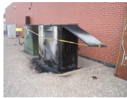
Auxiliary Transformer Seal (damaged)
