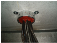
Cable Penetration Seal
