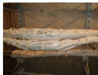
Cable Joint Wrap
