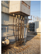
Transformer Cable Drop Penetration Seal
